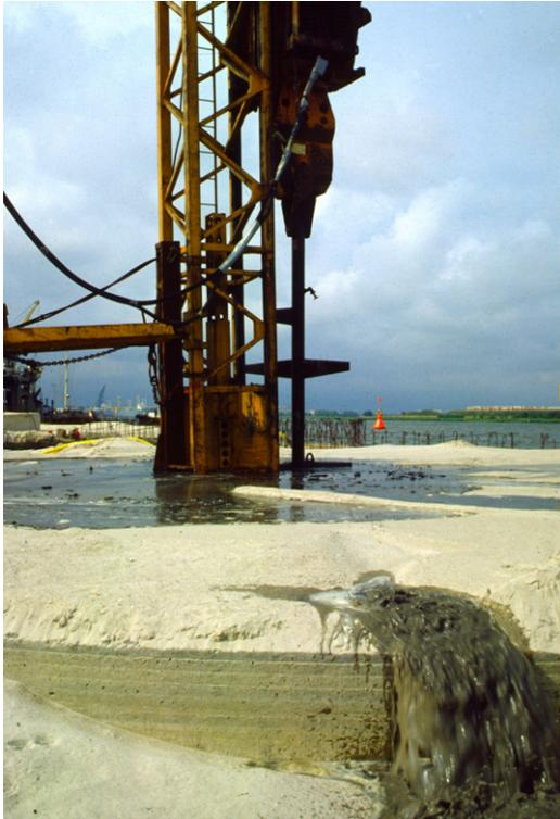
Figure 4. Water flow as evidence of liquefaction during compaction of the hydraulic fill inside the concrete caisson (source: Massarsch and Lindberg, 1984)
